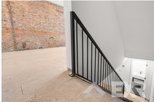
Ground Floor Entrance to Basement
